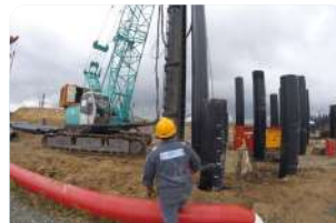
Jasa Pemancangan Piling Services
