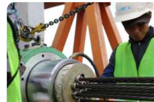
Jasa Stressing Post-Tension Post-Tension Stressing Services
